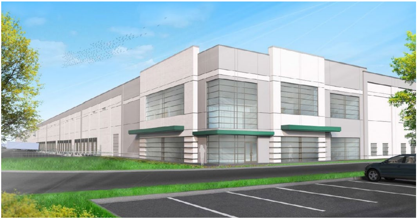
In June 2014, construction began on this 750,000-square-foot facility in Berks Park 78, an industrial park in Bethel Township, Penn.
